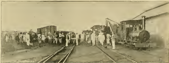
WORK ON A STATE ROAD IN INDIA.
